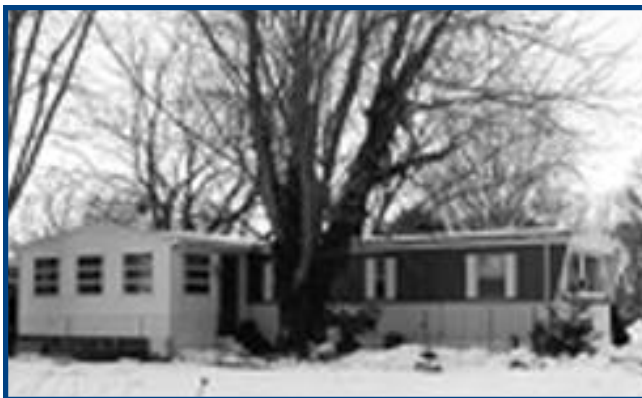
A manufactured home with a permanent addition. Green Acres Mobile Home Park.
