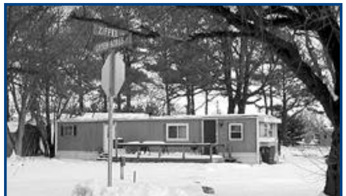
A manufactured home with a permanent deck attached. Green Acres Mobile Home Park.
